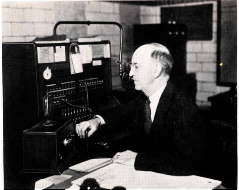
FIGURE 2—HAVERFORD TOWNSHIP POLICE DEPARTMENT. TRANSMITTER IS LOCATED IN CORNER OF ROOM WITHIN SIGHT OF OPERATOR, SEATED AT THE CONTROL BOX
