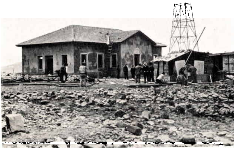
FIGURE 5—PROGRESS VIEW AT STATION CP3 AND CP4, LA PAZ.
